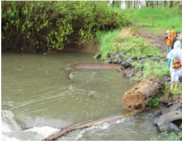
Figure 3 Upstream inlet of the culverts Image credit: Chris Gifford-Miears
