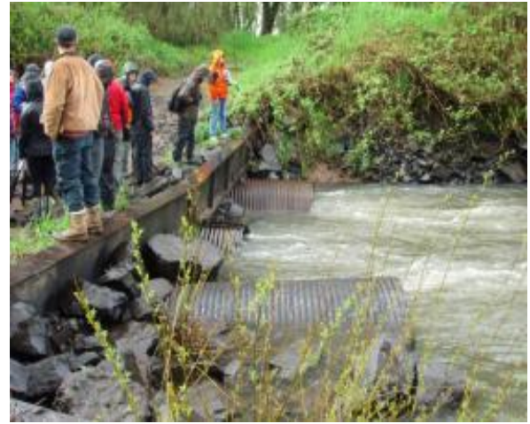
Figure 4 Downstream outlet of the culverts Image credit: Chris Gifford-Miears
