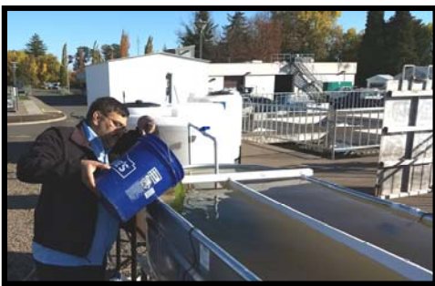
Dr. Ganti Murthy, Professor, seeds the bioreactor at the Corvallis Municipal Waste Water treatment facility with Chlorella .
